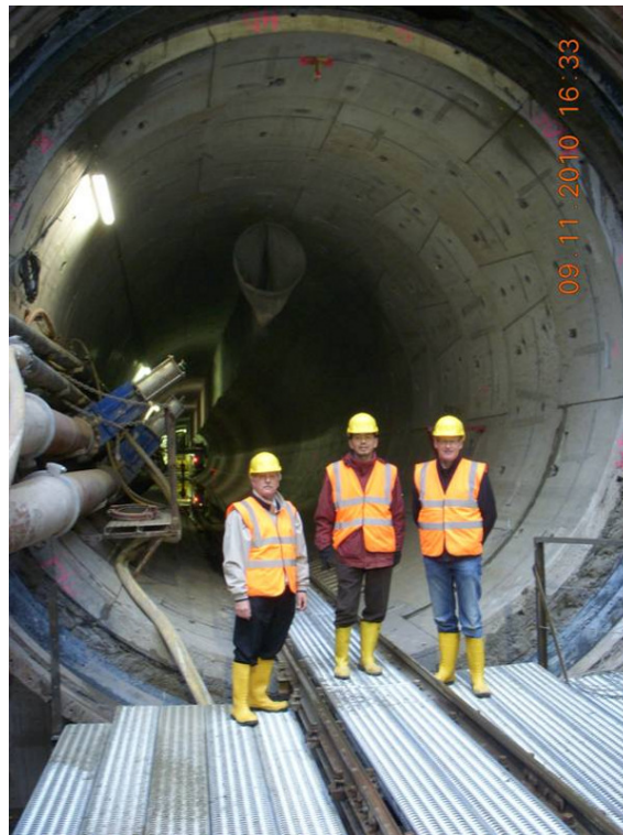
Figure 3: The three regional leaders from the civil facilities and siting (CFS) group after visiting the European XFEL tunnel boring machine in front of the tunnel mouth. The piping for the bentonite can be seen on the left. Image: John Osborne.
